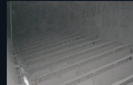
▲Inside of Silo (Cement Aeration System)
